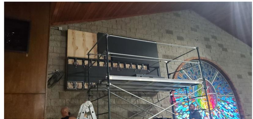
The cabinets will be mounted using lag screws, and the cabinets will be secured to one another using 3/8" nuts and bolts
